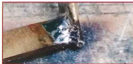
One of my soldered joints with way too much solder, but it can be Dremeled out.
